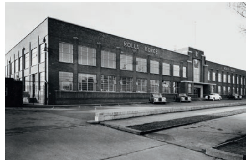
As part of the war effort, a new factory was built at Crewe in 1938 in a bid to increase the production of the Merlin engine. After the war, the motor division was transferred from Derby.
